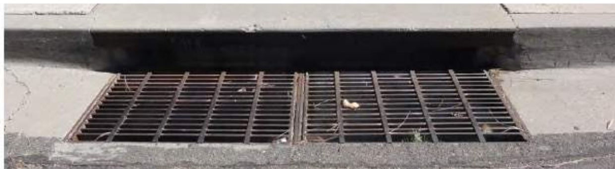
Storm Drain Inlet, Albuquerque, NM (photo by Tess Houle)
